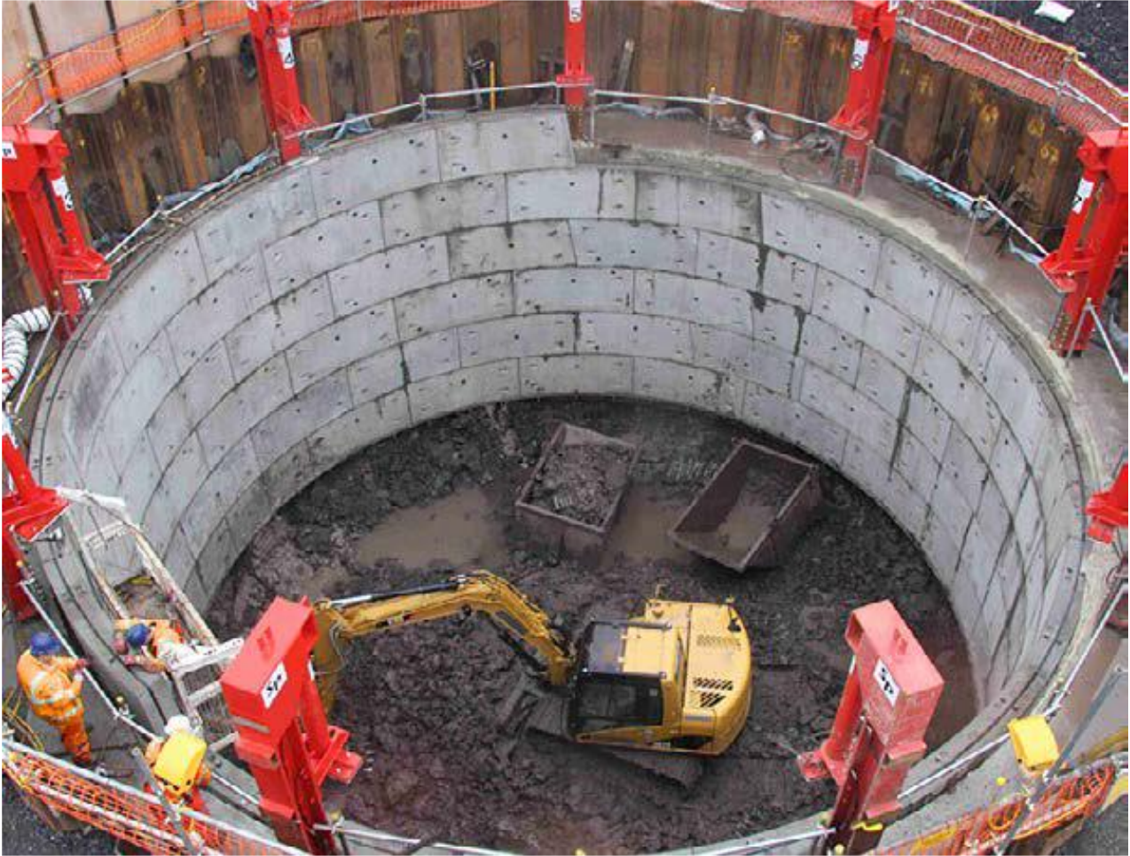
Graphic 2-10 Example of tunnel shaft construction
